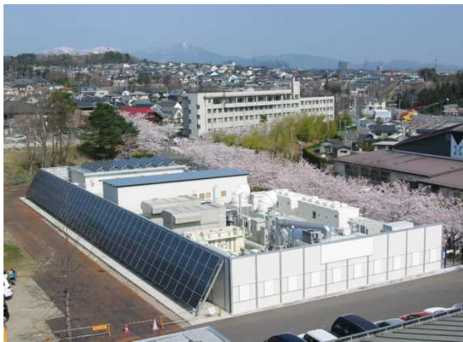
Sendai microgrid demonstration site in Japan
