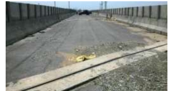
Access Road to Kamarajar Port
